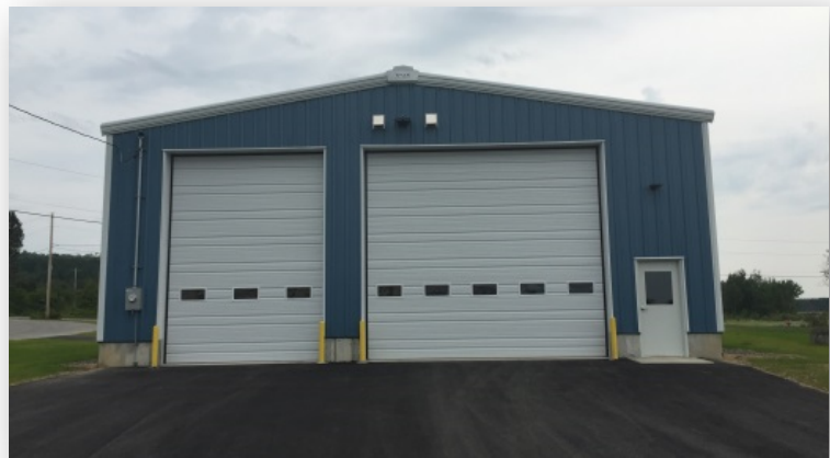
Figure 2.12 | Houlton's Snow Removal Equipment Storage Building
